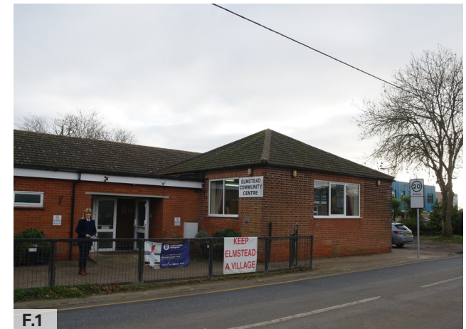
Figure 01: Existing village hall within Elmstead.
