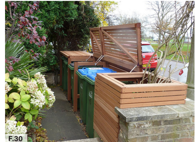
Figure 30: Waste storage along the boundary treatment.
